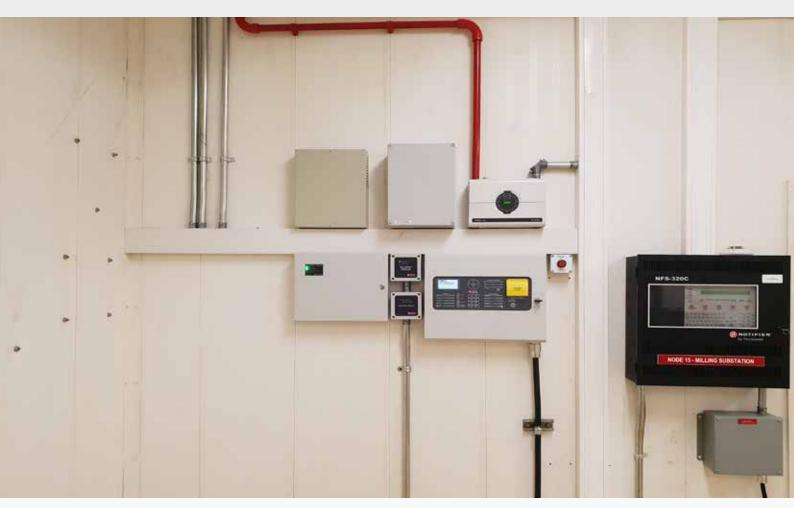
The FS Group developed and installed an ASD Early Warning Smoke Detection System combined with a pre-engineered FM200 Gas Suppression System with electrical actuation for 12 critical electrical infrastructure rooms.
