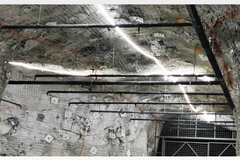
Keeping explosives underground in close proximity to operations poses a serious risk to the safety of miners. The FS Group has developed and installed a fully functional, quick response, electronically actuated Water Deluge system for an Underground Explosives Magazine. The system is designed so that all sprinklers in the area will discharge water in the event of a confirmed fire event, resulting in complete saturation of the entire area.
