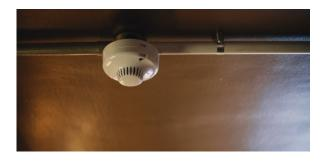
The first phase of the project was Fire Detection which included replacing wireways, upgrading **13000 meters of cable**, installing Fire Panels, **1200 Smoke Detectors and 70 break glass units**.
