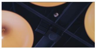
For the public address system, a total of 48 speakers were installed. The Theatre has many big open spaces, so typical speakers could not be installed. Due to the acoustic ceiling in the Foyer, which absorbs sound, the speakers had to be set up accurately to get sound down into the foyer. Cluster based speakers were chosen and suspended about 20 meters up in the air, so that they did not affect the ascetics.
